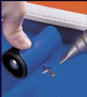
Welding a patch on a tarp
